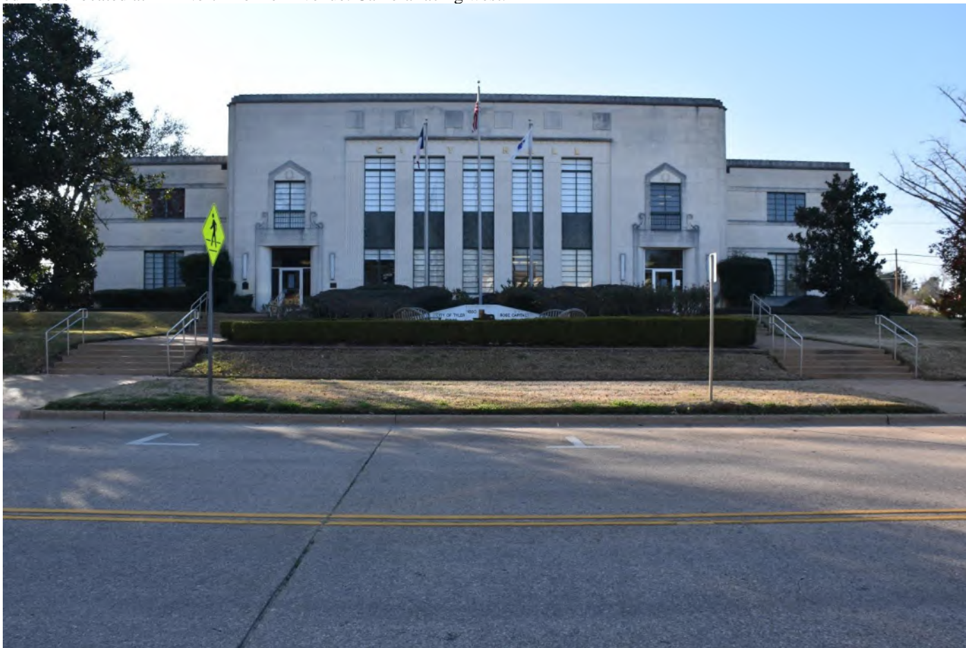
Photo No. 38. View of Tyler City Hall (Resource 19), showcasing Classical Revival and Art Deco stylistic influences. The 1938 edifice is located at 212 North Bonner Avenue. Camera facing west.
