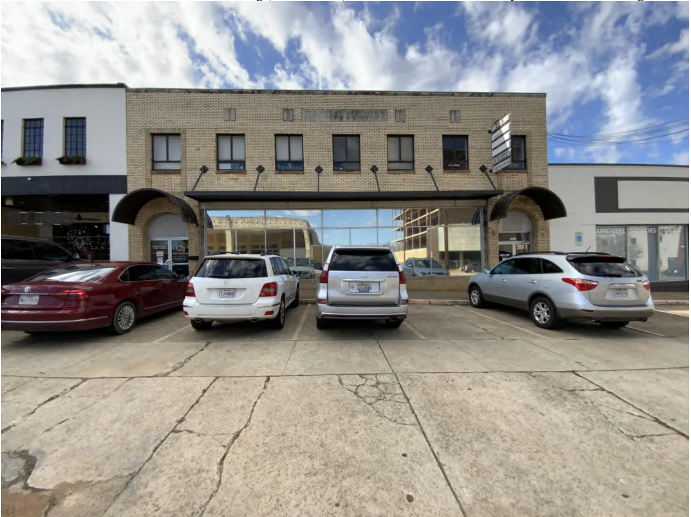
Photo No. 49. View of the 1938 Manziel Building (Resource 108), located at 235 South Broadway Avenue. Camera facing west.
