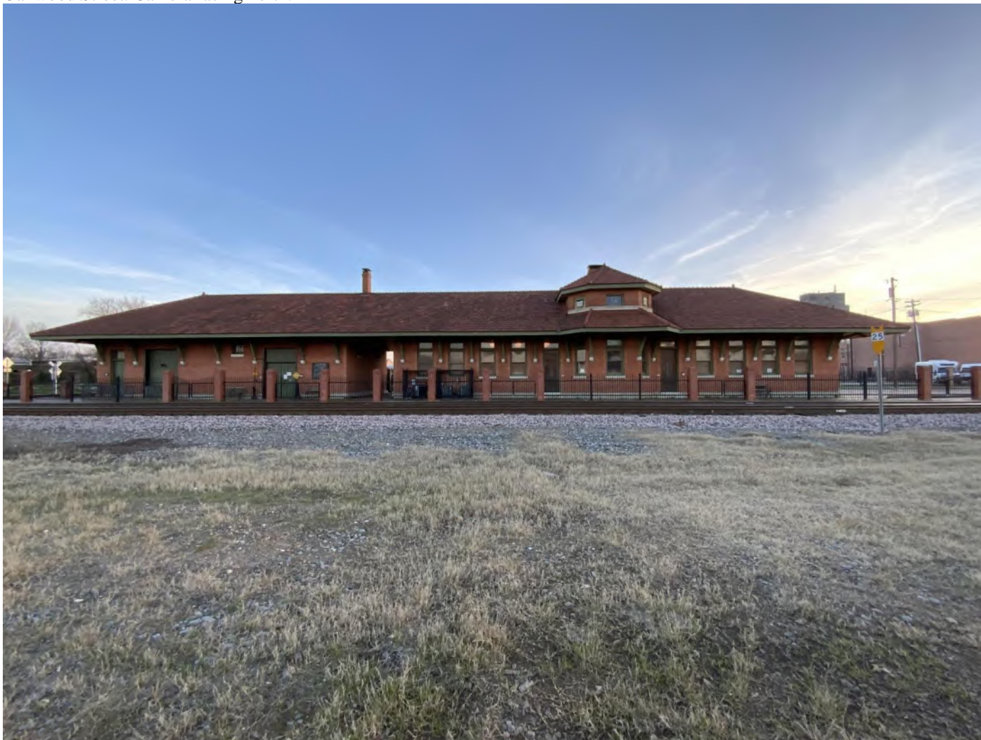
Photo No. 18. View of the St. Louis Southwestern Railway (Cotton Belt) Passenger Depot (Resource 2), located at 210 East Oakwood Street. Camera facing north.
