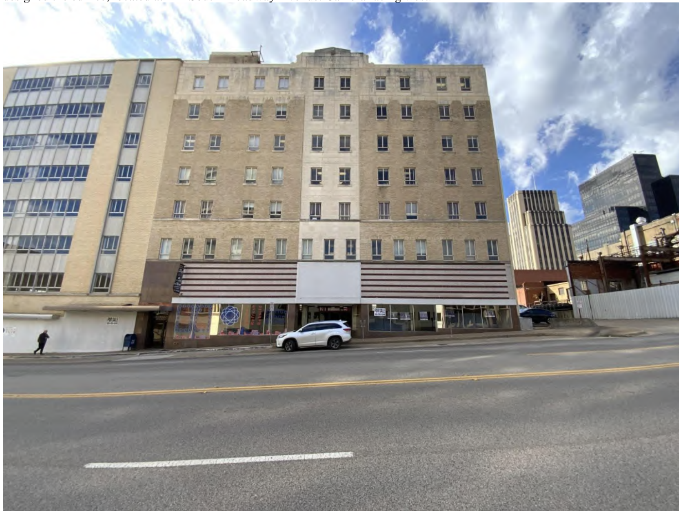
Photo No. 39. View of the Fair Foundation building (Resource 96), constructed in 1949. Jacksonville-based architect S.W. Ray designed the edifice, located at 121 South Broadway Avenue. Camera facing west.
