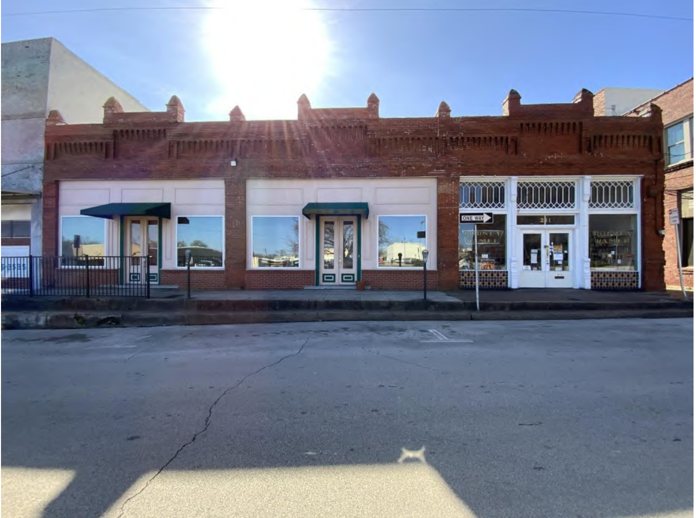
Photo No. 16. Frontal view of the Kamel Building (Resource 50), located at 211-215 East Ferguson Street. Camera facing northwest.
