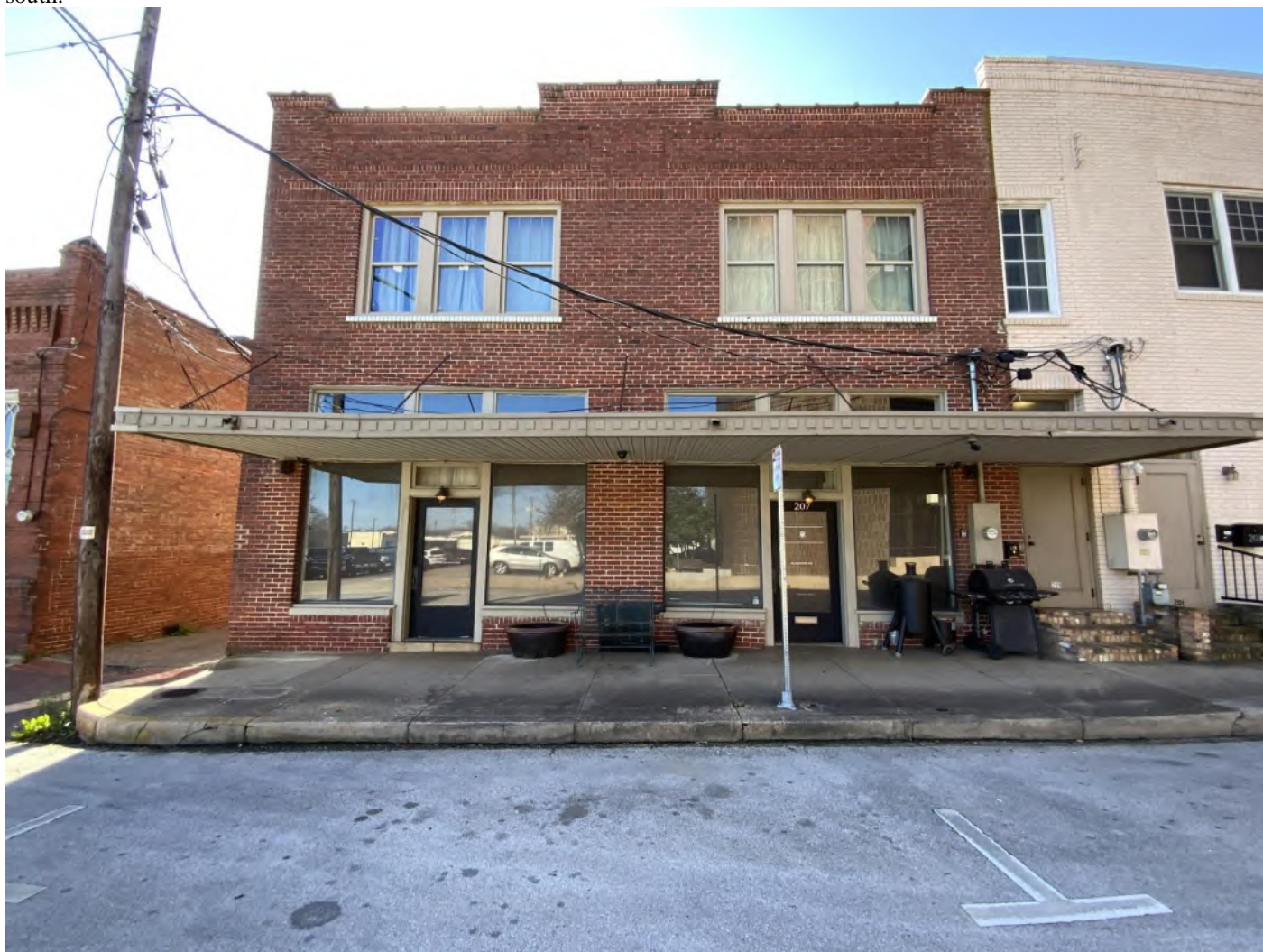
Photo No. 47. View of a two-part commercial block building (Resource 59), located at 207-209 East Ferguson Street. Camera facing south.
