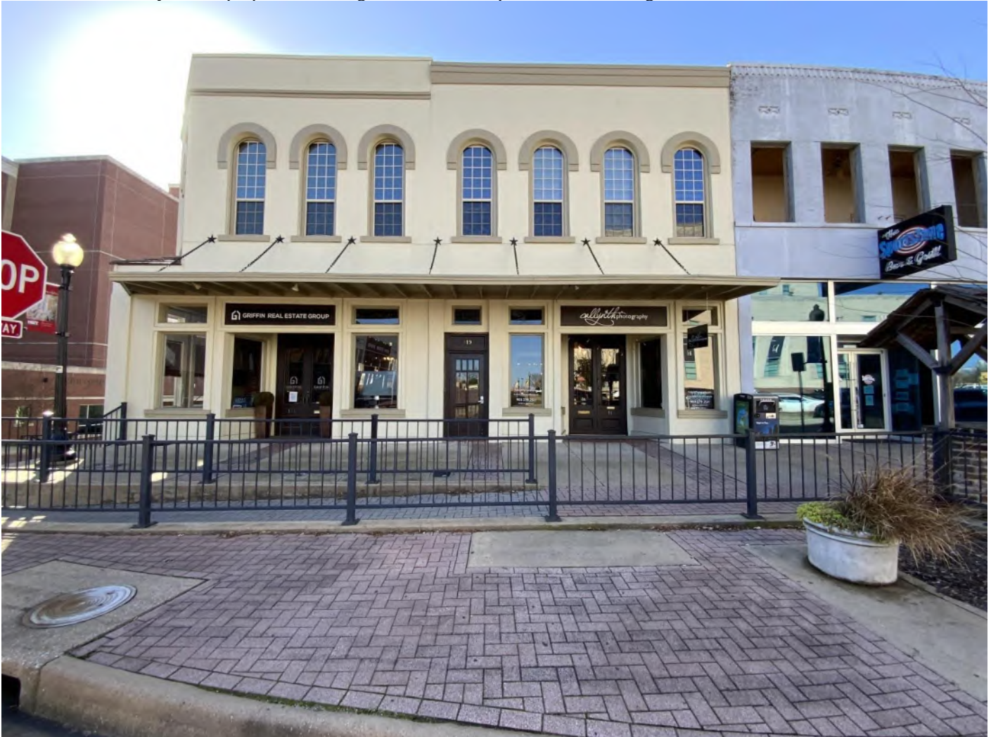
Photo No. 53. View of the two-part commercial block building (Resource 84) located at 117-121 West Erwin Street, an example of one of the extensively altered properties fronting the courthouse square. Camera facing south.
