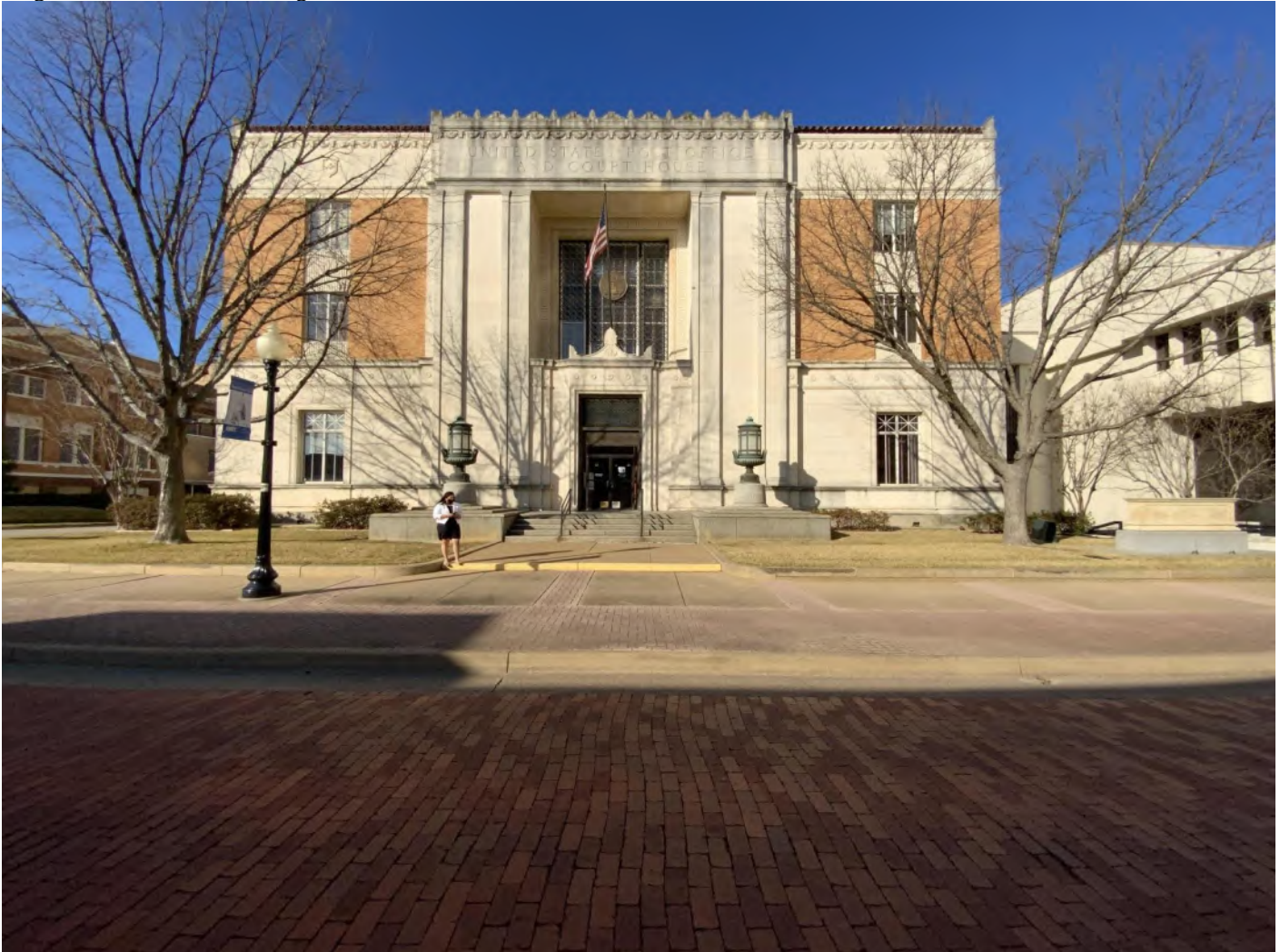
Photo No. 35. View of the Tyler U.S. Post Office and Courthouse/Tyler Federal Building (Resource 36) located at 221 West Ferguson Street. Camera facing north.
