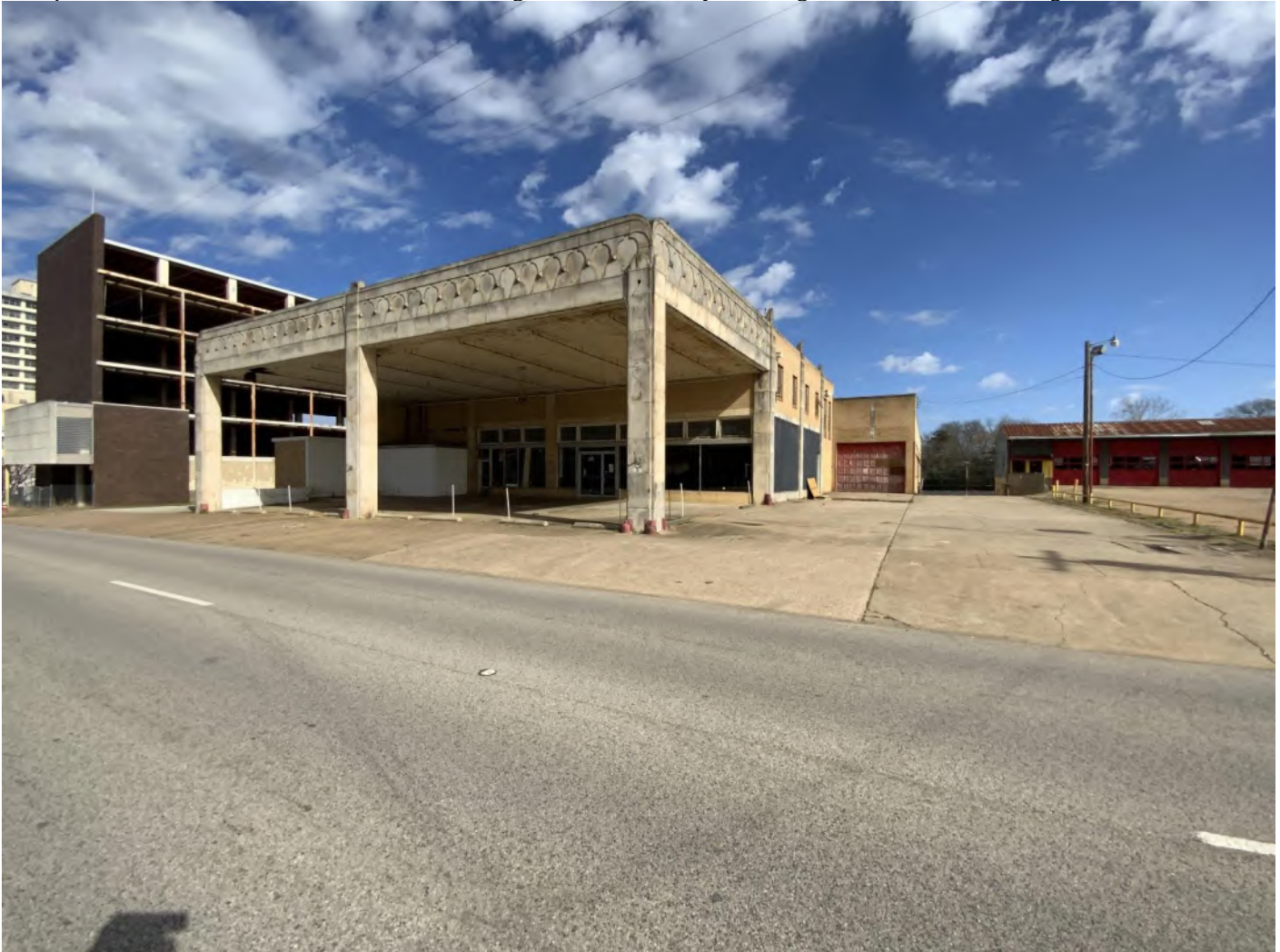
Photo No. 33. Oblique view of the Holley Motor Company building (Resource 110), located at 236 South Broadway Street, another example of an automobile-related business that emerged in downtown Tyler during the 1930s. Camera facing northeast.
