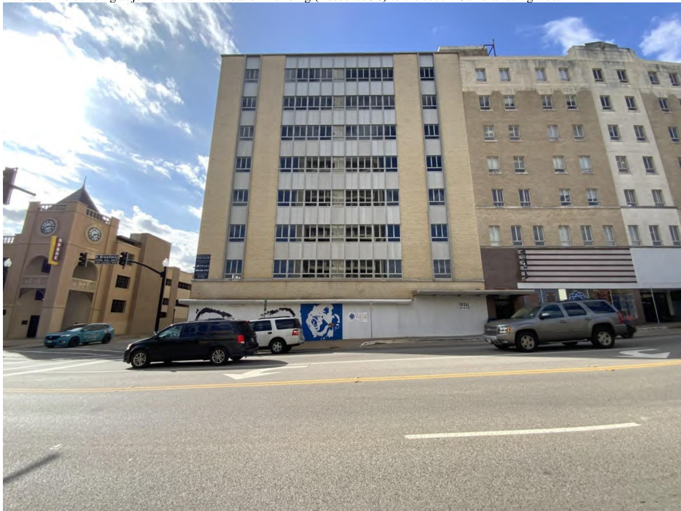
Photo No. 40. View of the 1954 S.A. Lindsey Building/Fair Petroleum Building (Resource 99), located at 115 South Broadway Avenue. The building adjoins the Fair Foundation Building (Resource 96) to the south. Camera facing west.
