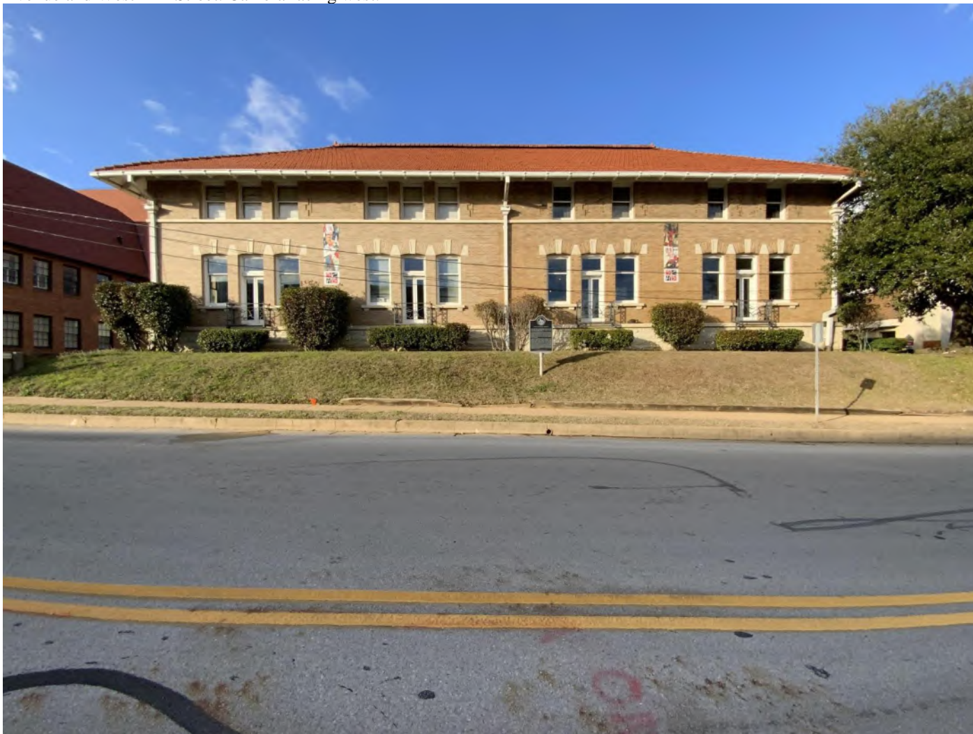
Photo No. 19. View of the side façade of Tyler Carnegie Library (Resource 94), located at the northwest corner of South College Avenue and West Elm Street. Camera facing west.
